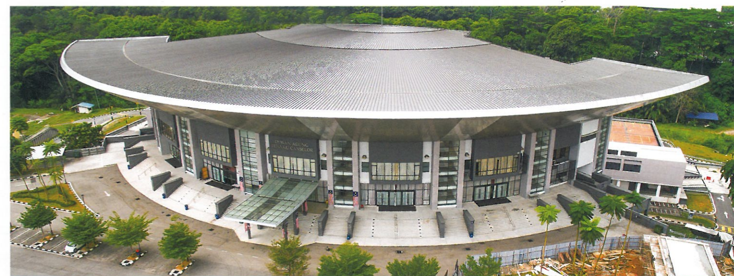
UiTM Shah Alam Campus, Dewan Agung - Shah Alam, Selangor - Roofing
