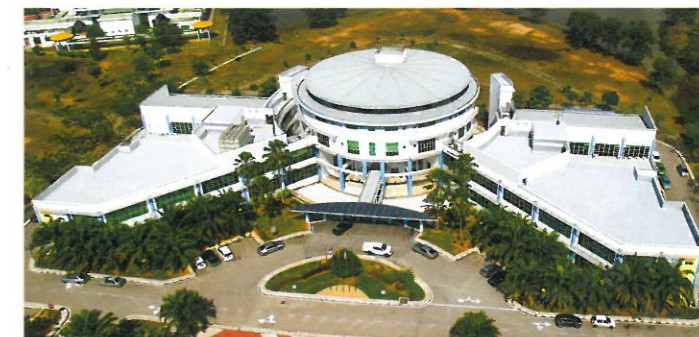
University Industri - UNISEL, Bestari Jaya, Selangor - Roofing
