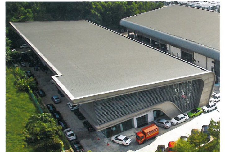
Wing Hin Autohaus (Volkswagen) - Balakong, Selangor - Wall Cladding & Roofing.
